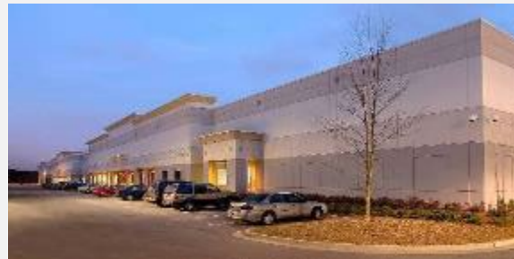
Airport West Distribution Center, Atlanta, GA
